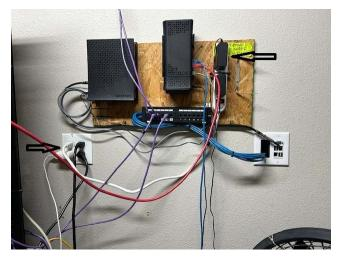
We have two UPS units in the server room. The one in the system cabinet powers the power distribution strips along the side of the cabinet. These accept special NEMA 13 type power cords. The Spectrum modem and its partner unit have regular computer cords with NEMA 15 110v ends. We have other devices with NEMA 15 cords, and thus had an additional UPS (Cyberpower CP550SLG) on the floor to support them.
